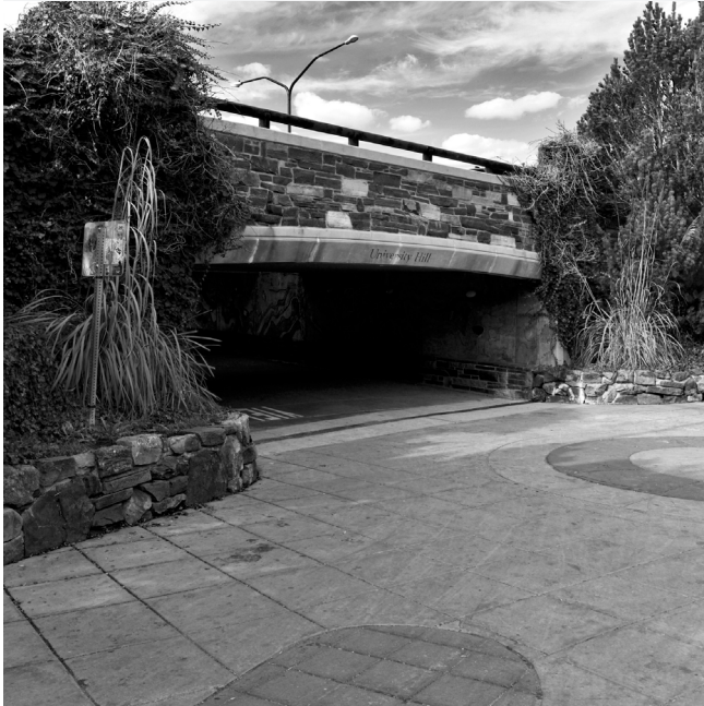
Figure 5. The Broadway underpass at College Avenue, which connects the CU Boulder campus to the University Hill commercial area.
